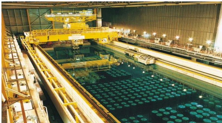
Figure 2. A pond for used nuclear fuel at the Sellafield waste processing center, sourced from the World Nuclear Association ( Radioactive Waste Management - World Nuclear Association (world-nuclear.org) )
